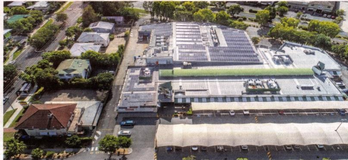
BETTER FOR ALL: An aerial view of Noosa Village shopping centre with solar array.
