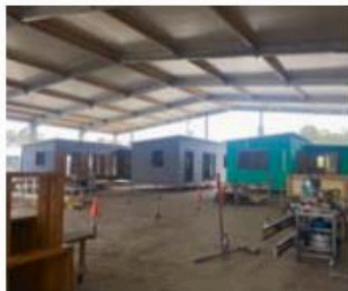
Eco-Cottages in production.
