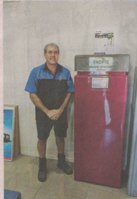
Andrew Chapman with battery system.
